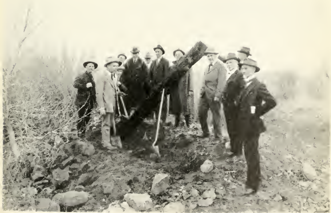
EXCAVATING A LOG (NOVEMBER 9, 1922) THAT FORMED A PORTION OF THE CRIBBING FOR ONE OF THE PIERS OF OLD PLATTE BRIDGE. BUILT IN 1858-9.
