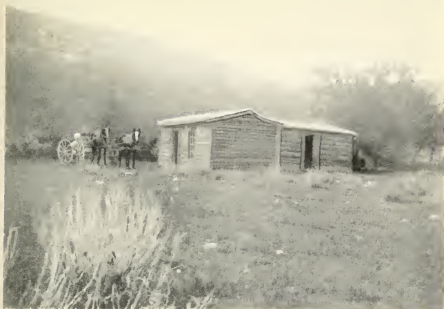
THE "HOLE-IN-THE-WALL" CABIN
