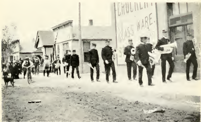
CASPER BAND MARCHING DOWN CENTER STREET, 1908 Buildings on east side, from left to right: Trevett's store, Norton & Hagens' law office, Tribune office, Webel's store.
