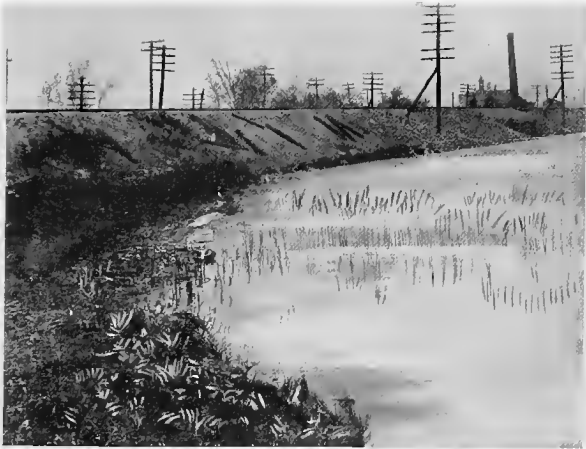
FIG. 8 —Railroad crossing Cochituate Lake from which comes part of the water supply of Boston. The drainage from the tracks is directly into the lake.
